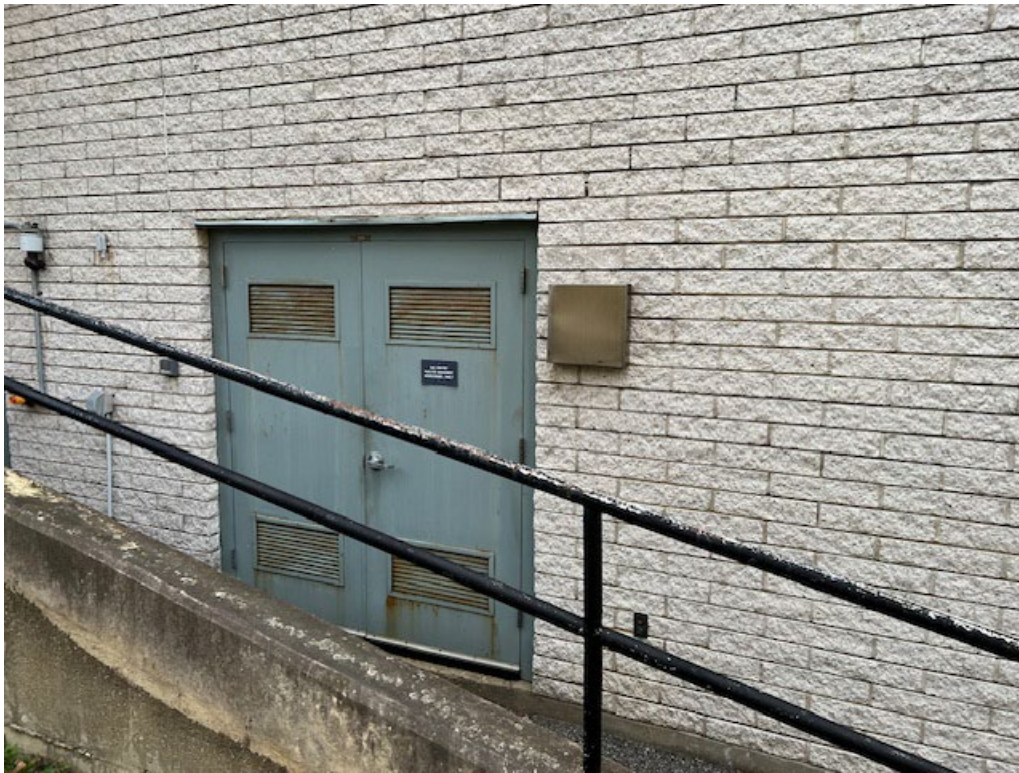
Exterior access to Mech/Elec Room - Basement
