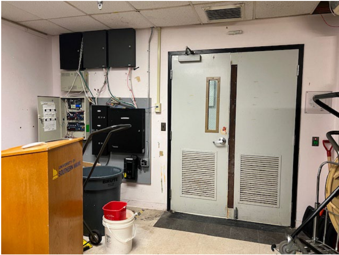
Interior views of Storage Room – Ground Floor
